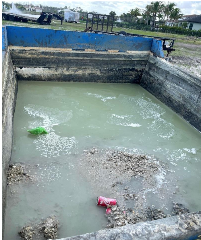
Figure 7-5. Concrete washout container filled with some contaminants.
