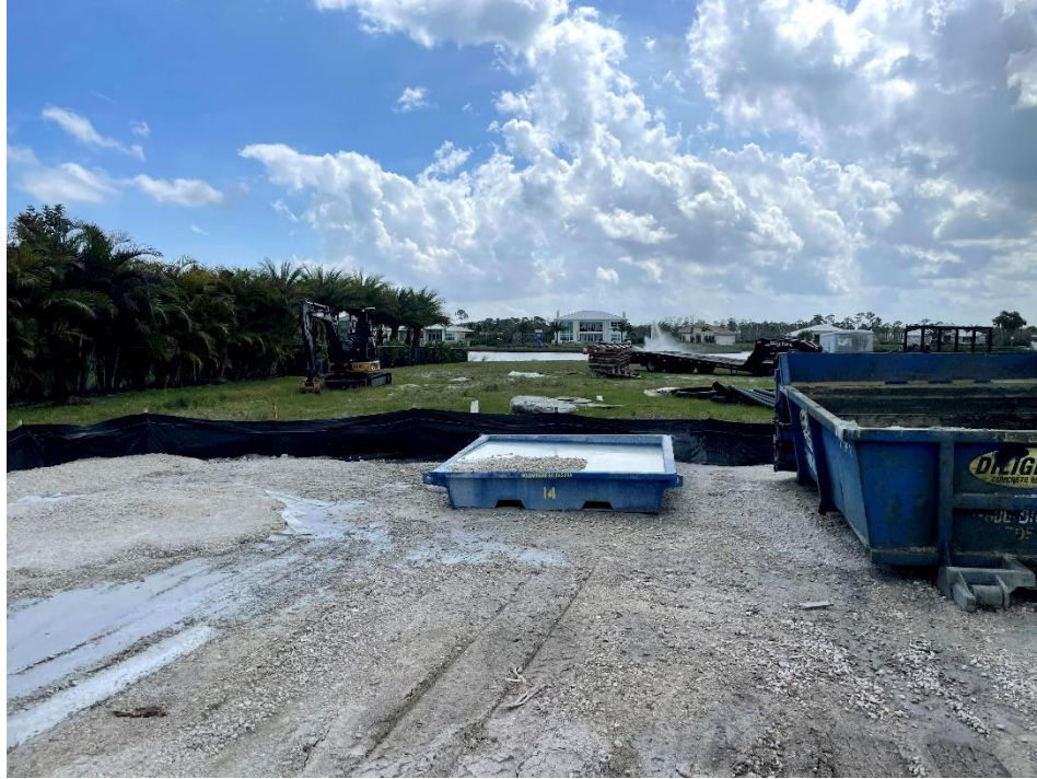
Figure 7-4. Concrete washout placed on ground and placed in best management container.
