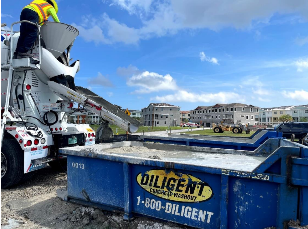
Figure 2-2. Concrete ready-mix truck operator washing out chute and truck.
