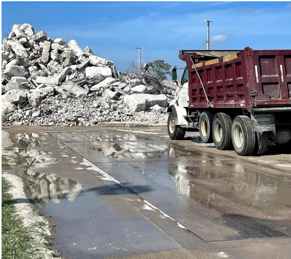
Figure 7-7. Concrete washout recycling facility where it is crushed and used/reused as aggregate for new concrete.
