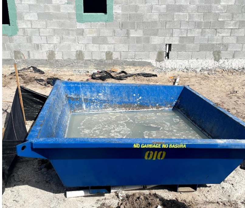
Figure 7-6. Concrete washout collection container in a construction site with limited space.
