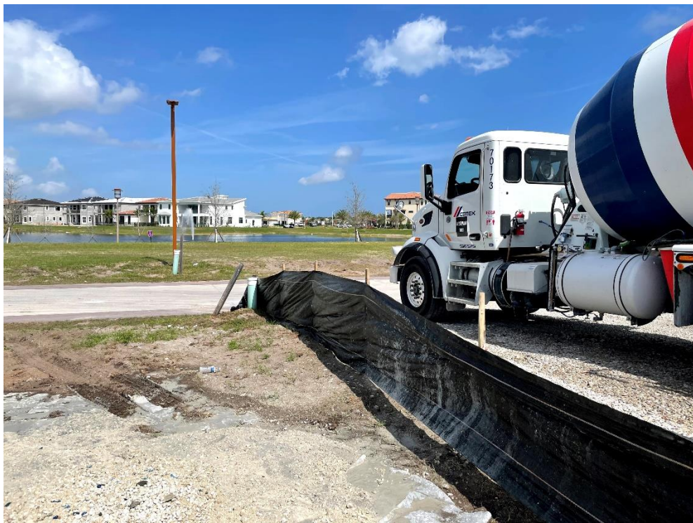
Figure 7-1. Concrete washout directly placed on tarp on ground.
