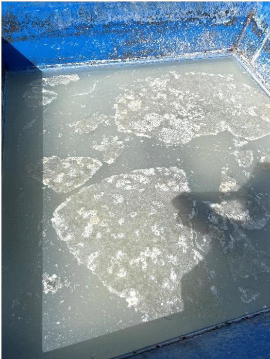
Figure 2-3. Concrete washout collected.
